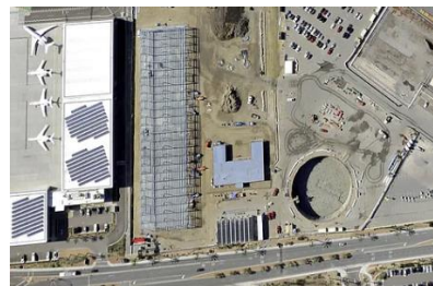
Construction of a 3 million-gallon cistern at San Diego International Airport
