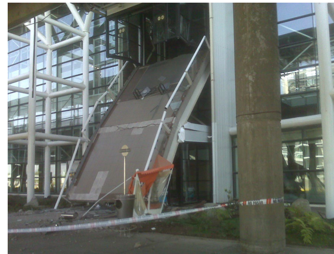
Santiago: 8.8 M_w , 27 Feb 2010. Airport pedestrian bridge
